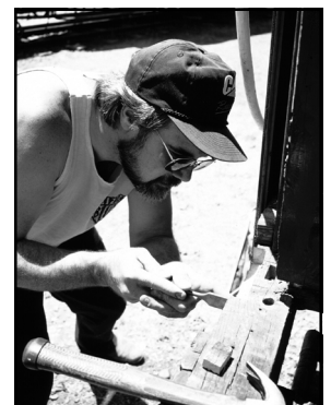
Duane Fields trimming a mortise with a chisel. Photo © Steve Mason
